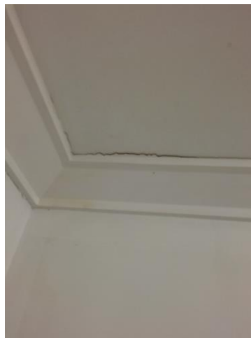
Cornice cracking
