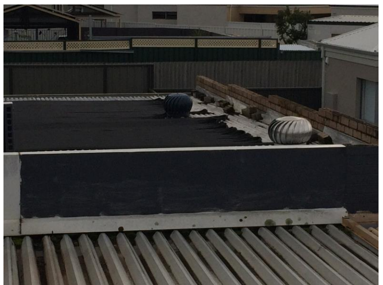
Flashing material and installation incorrect
