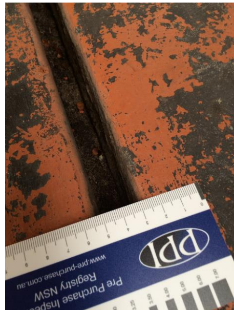
Driveway separation at control joint
