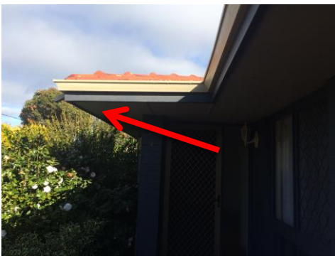
Front Hip dips to this external corner
