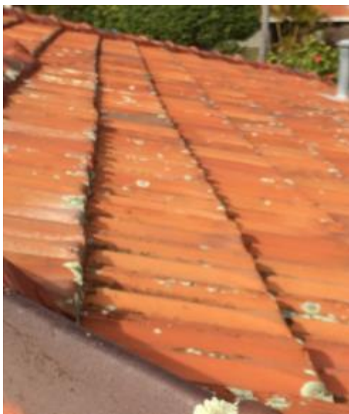
Undulating roof cover
