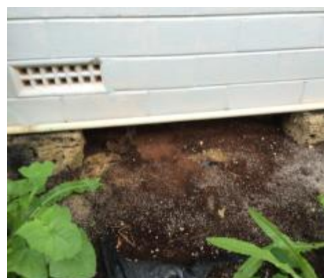
Sub Floor Access Blocked
