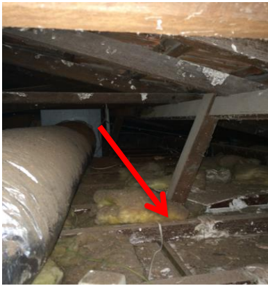
Insulation displaced in areas
