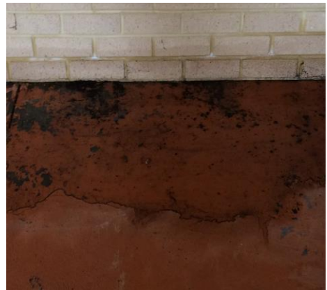
Inadequate drainage causing rising damp, rear garage
