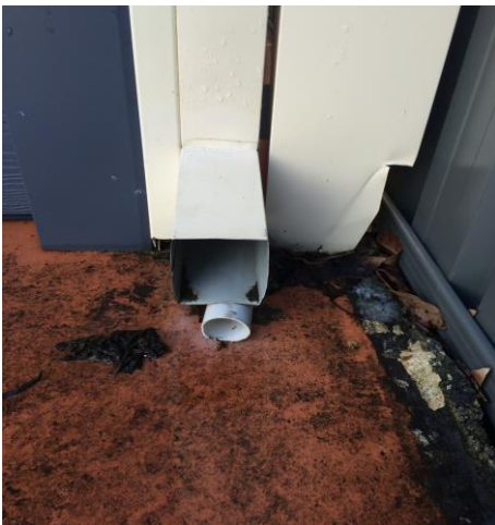
Inadequate stormwater disposal
