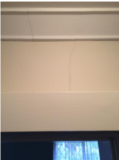
Cornice/Wall cracking
