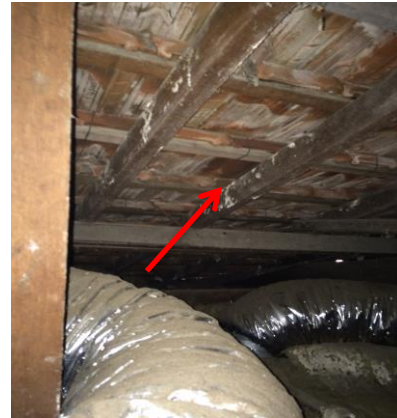
Evidence of water penetration
