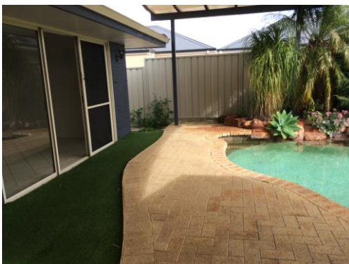
External site level higher than internal floor area, Inadequate drainage issues
